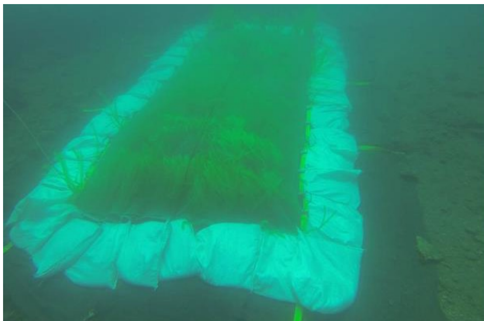
Fig. 19: Artificial seagrass mat. Sandbags are placed on the apron around the mat to keep it in place. Photo Nationalmuseet
