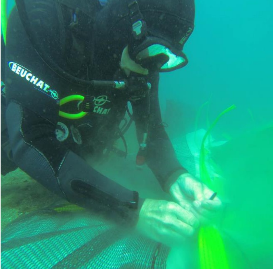
Fig. 20: The apron is secured around the sandbag to keep the mat in place Photo Nationalmuseet
