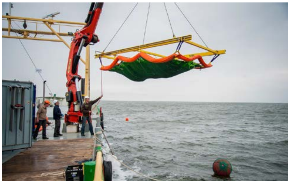
Fig. 14: The artificial seagrass being deployed on the wreck of BZN10. Photo Paul Voorthuis
